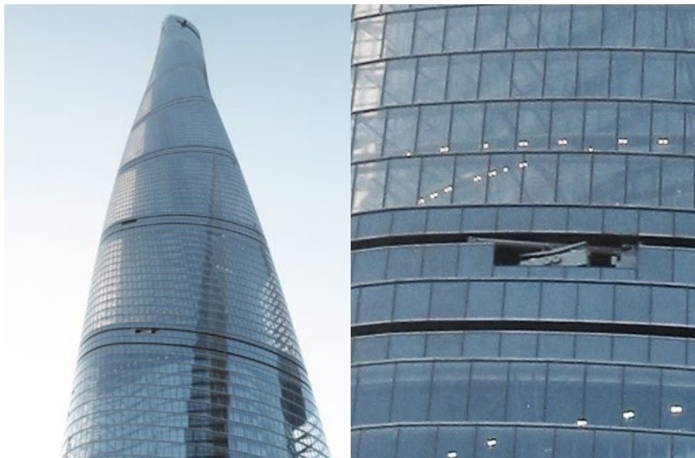
Shanghai Tower: 3D climbing building maintenance unit capable of changing climbing angle and traversing direction at the same point on the track
