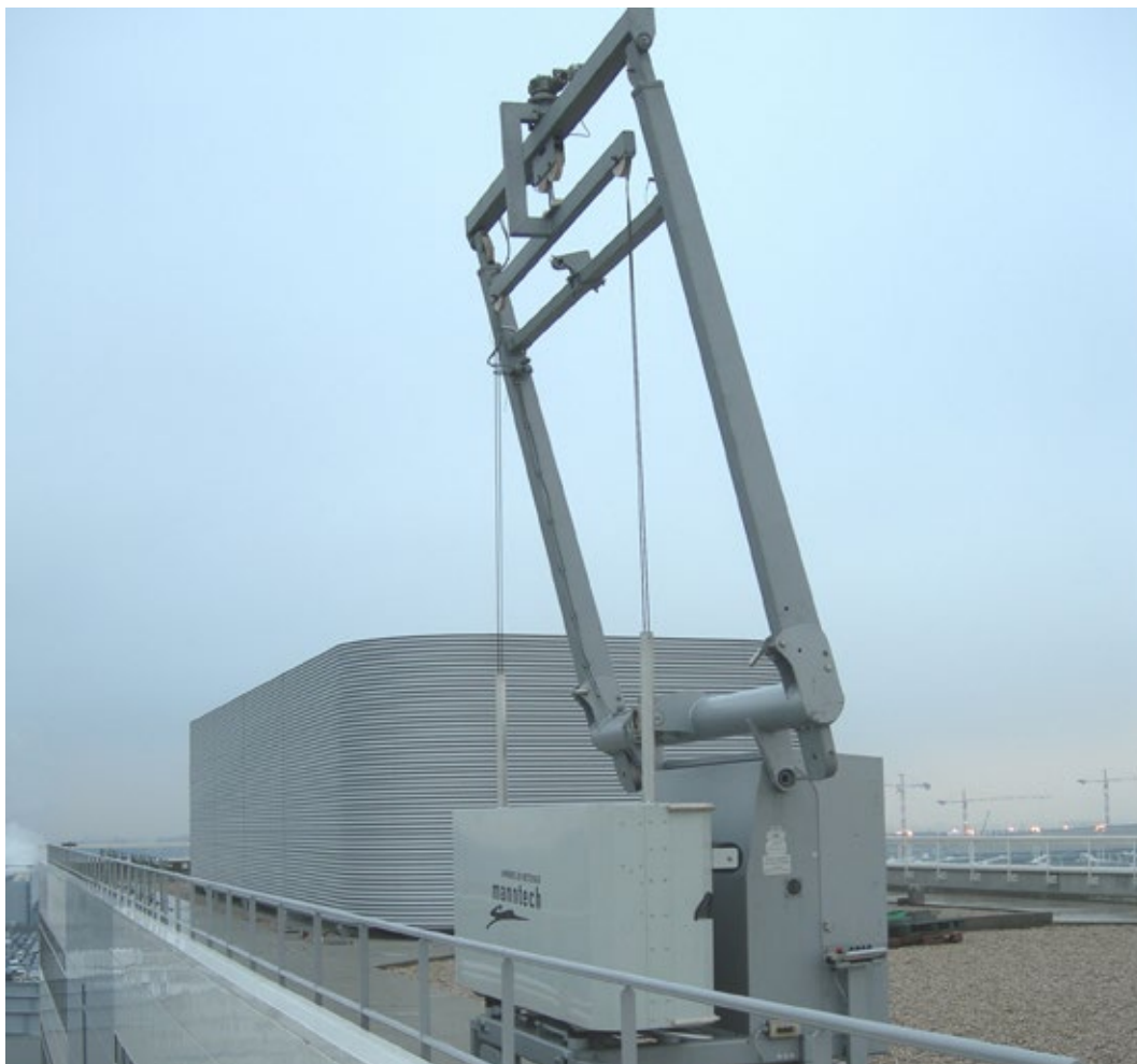
Type 1.3 with crossbar for load-bearing hoist
