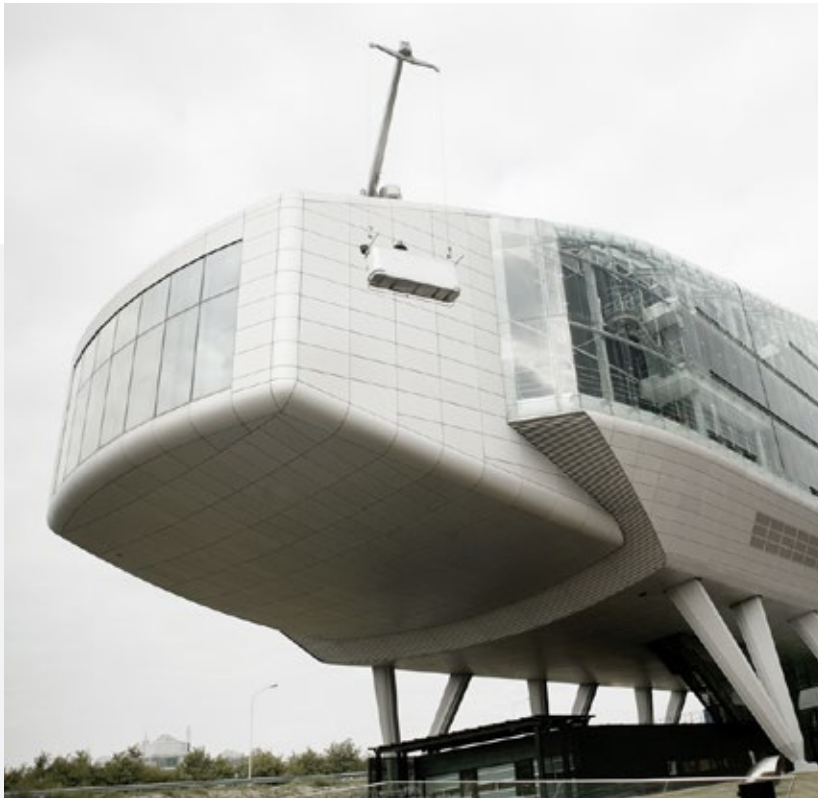
ING Bank, Amsterdam: Sloped track sections with a Type 6.1 BMU, here with rack and pinion drive and slewing head in a special design.
