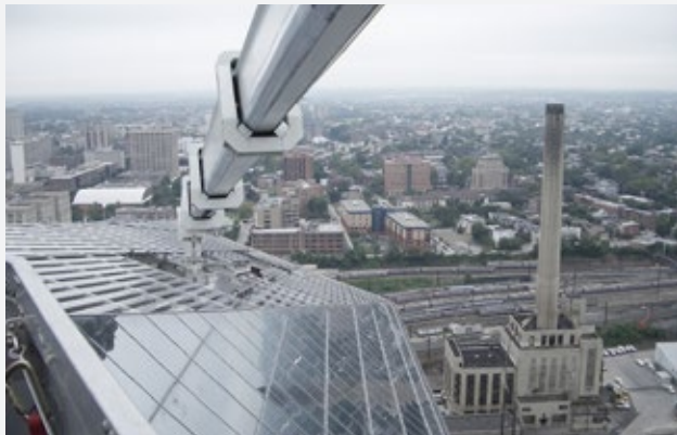
Type 6.1 with a quadruple telescopic jib and a vertical telescopic mast, completely retractable on the roof.
