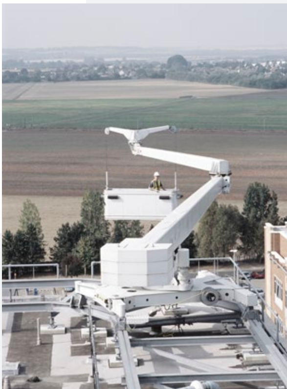
Type 6.1 track-based with horizontal slewing articulated jib
