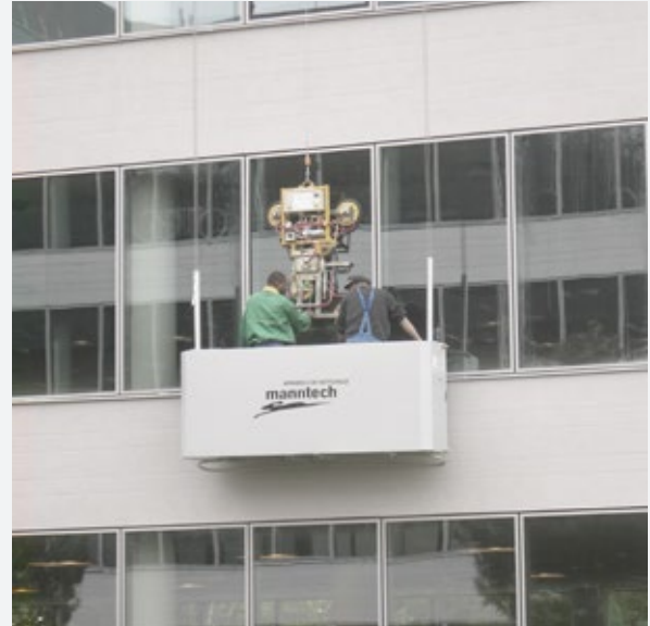
▶ Auxiliary hoist to transport glass panels and elements outside the cradle
