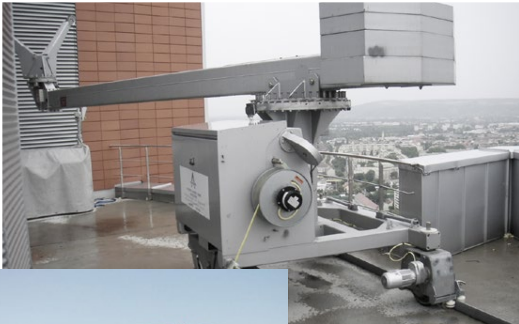
Type 4.3 with guide rail on the roof
