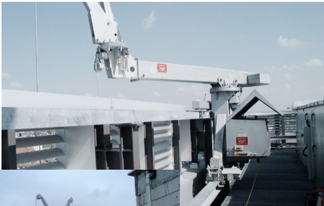
Type 4.2 low profile design with high V-head
