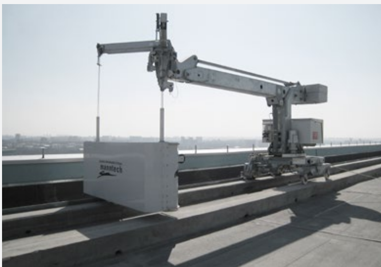
Type 6.3 with luffing jib and coupling bar for slewing head alignment
