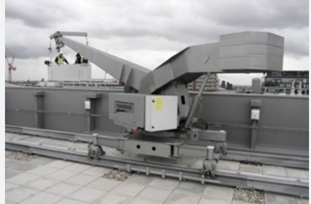
Type 6.2 track-based with fixed luffing jib, low-profile design.
