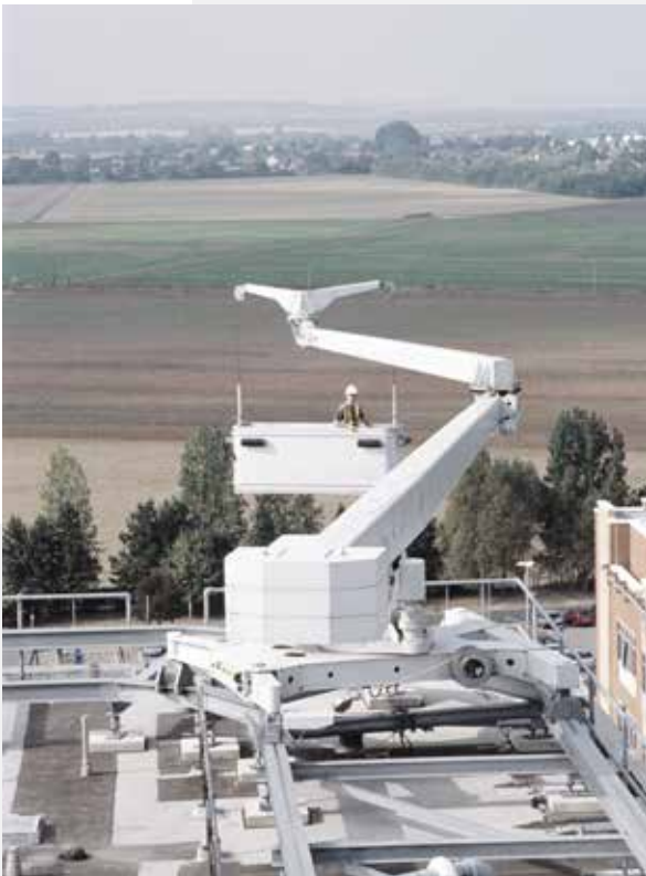
Type 6.1 track-based with horizontal slewing articulated jib
