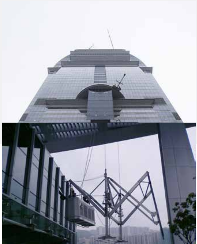
Various cantilevered cradle solutions for reaching recesses in building
