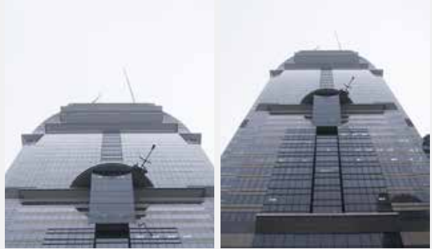
Type 6.1 triple telescopic jib and a satellite cradle for reaching recesses on the facade.
