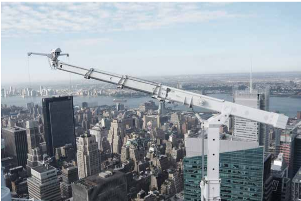
Crane BMU with telescopic jib
