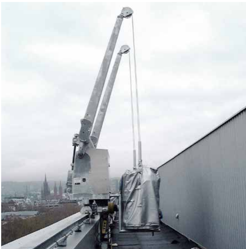
Type 1.2 in parked position with covered work platform
