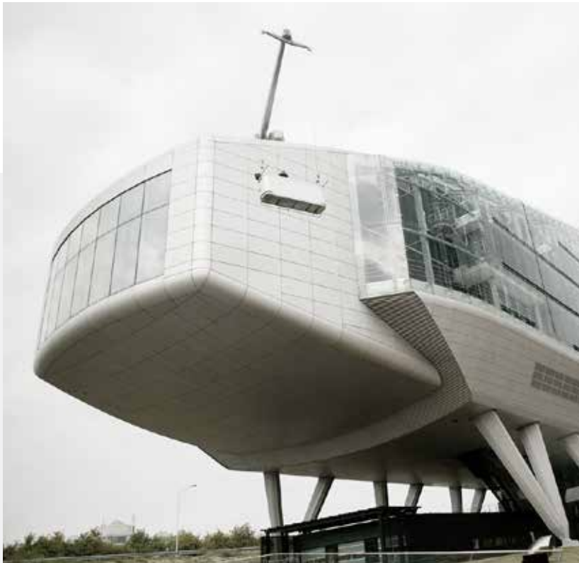
ING Bank, Amsterdam: Sloped track sections with a Type 6.1 BMU, here with rack and pinion drive and slewing head in a special design.
