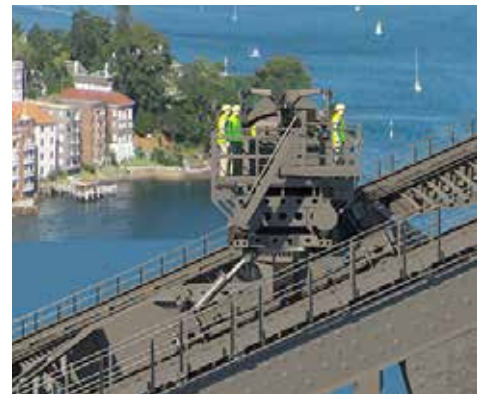
Sydney Harbour Bridge: Custom gantry-based bridge access system
