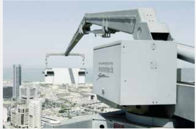
Type 6.1 track-based with vertical slewing articulated jib to reach recessed building areas
