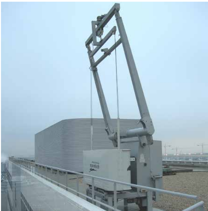
Type 1.3 with crossbar for load-bearing hoist
