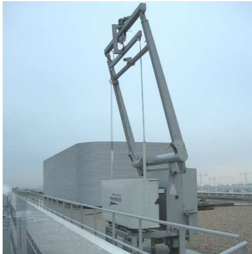
Type 1.3 with crossbar for load-bearing hoist
