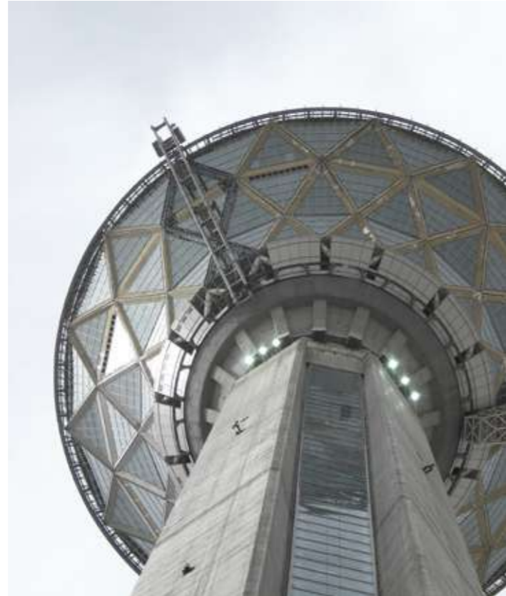
Milad Tower, Iran: Sloped elevator for maintenance of tower cupola. Designed for extreme wind stress and seismological conditions.
