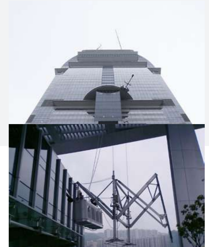
Various cantilevered cradle solutions for reaching recesses in building
