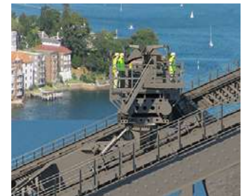
Sydney Harbour Bridge: Custom gantry-based bridge access system
