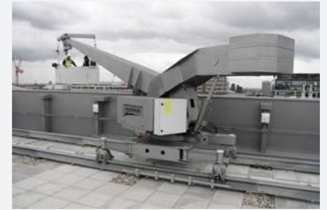
Type 6.2 track-based with fixed luffing jib, low-profile design.
