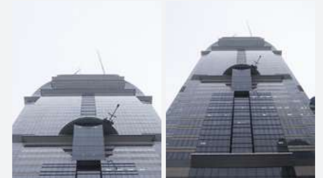
Type 6.1 triple telescopic jib and a satellite cradle for reaching recesses on the facade.
