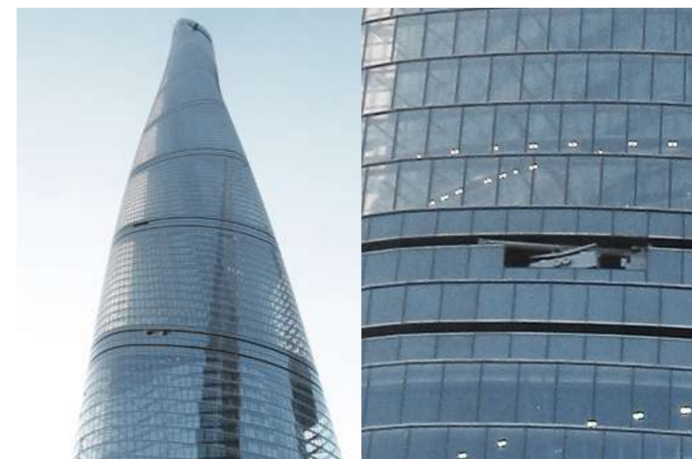
Shanghai Tower: 3D climbing building maintenance unit capable of changing climbing angle and traversing direction at the same point on the track
