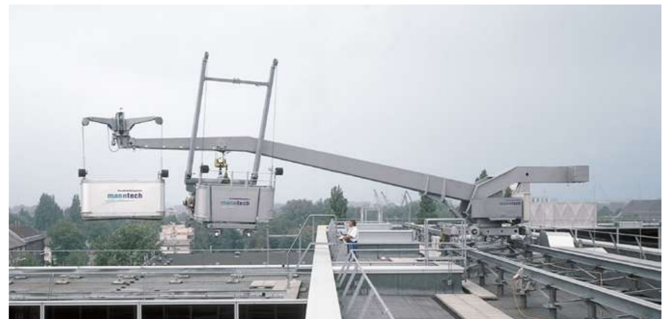
Type 6.1 track-based with fixed luffing jib and mechanism (load-bearing hoist) for transportation of a Type 1.1 BMU to various parts of the building.
