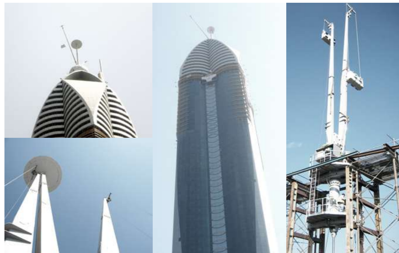
Rose Rotana Hotel, Dubai: Retractable crane BMU with twins jibs for optimal cleaning service
