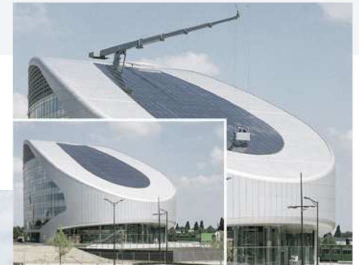
Type 6.4 stationary with a quadruple telescopic jib (BMU is completely retractable on the roof).
