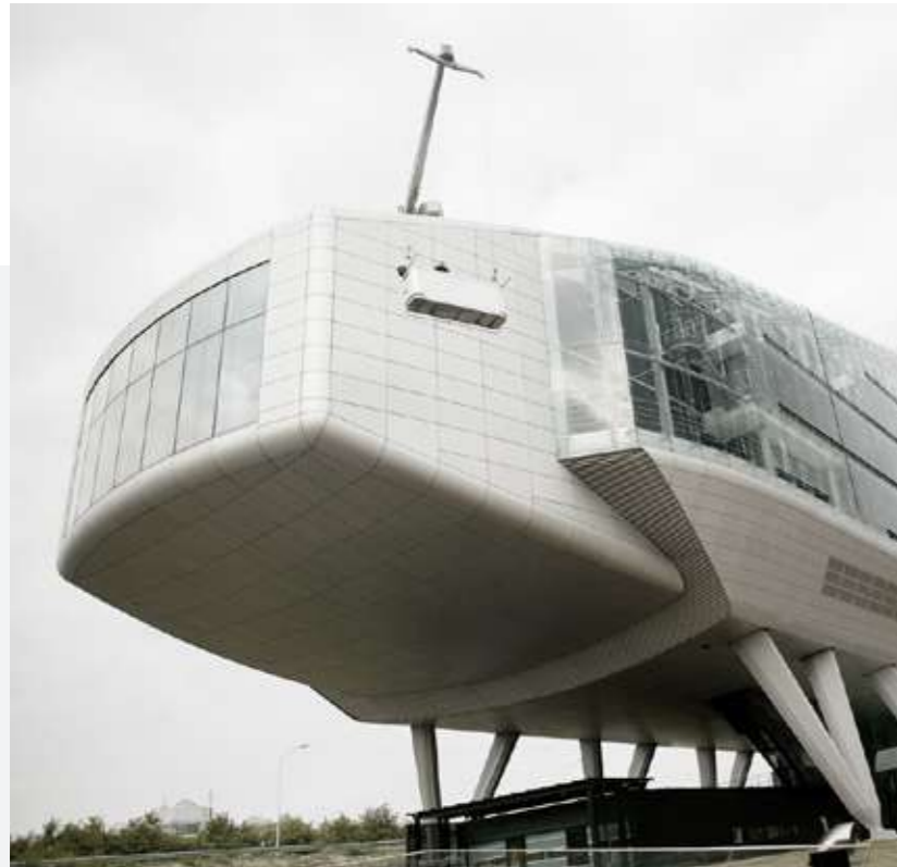
ING Bank, Amsterdam: Sloped track sections with a Type 6.1 BMU, here with rack and pinion drive and slewing head in a special design.
