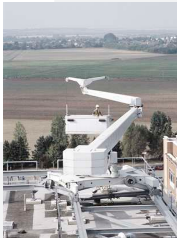
Type 6.1 track-based with horizontal slewing articulated jib
