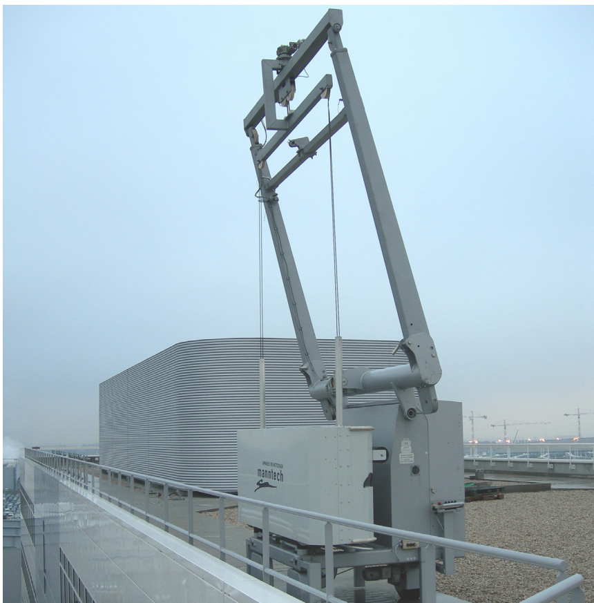
Type 1.3 with crossbar for load-bearing hoist
